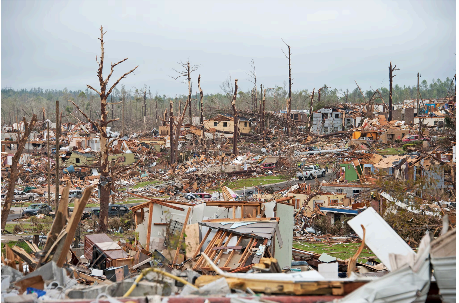
EF5 Tornado Damage, Birmingham, Alabama, 2011.
